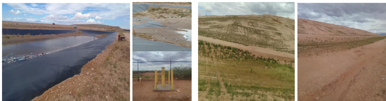
Figure 2.7. Components of Corralitos on-site contaminant management system: L-R: Leachate in lined evaporation pond; vadose well used to monitor groundwater; vegetative cover being installed on closed cell to manage erosion of sediments.
