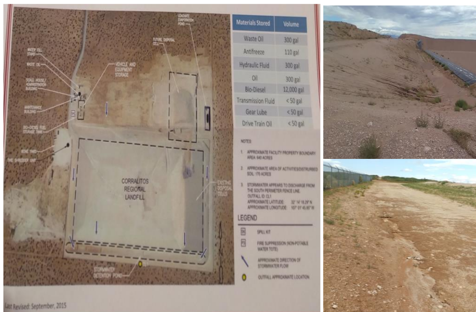
Figure 2.8. Illustration of stormwater flow, detention pond, discharge outfall, and water erosion at Corralitos.
