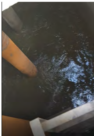
Photograph 9: Water level inside of wet well
