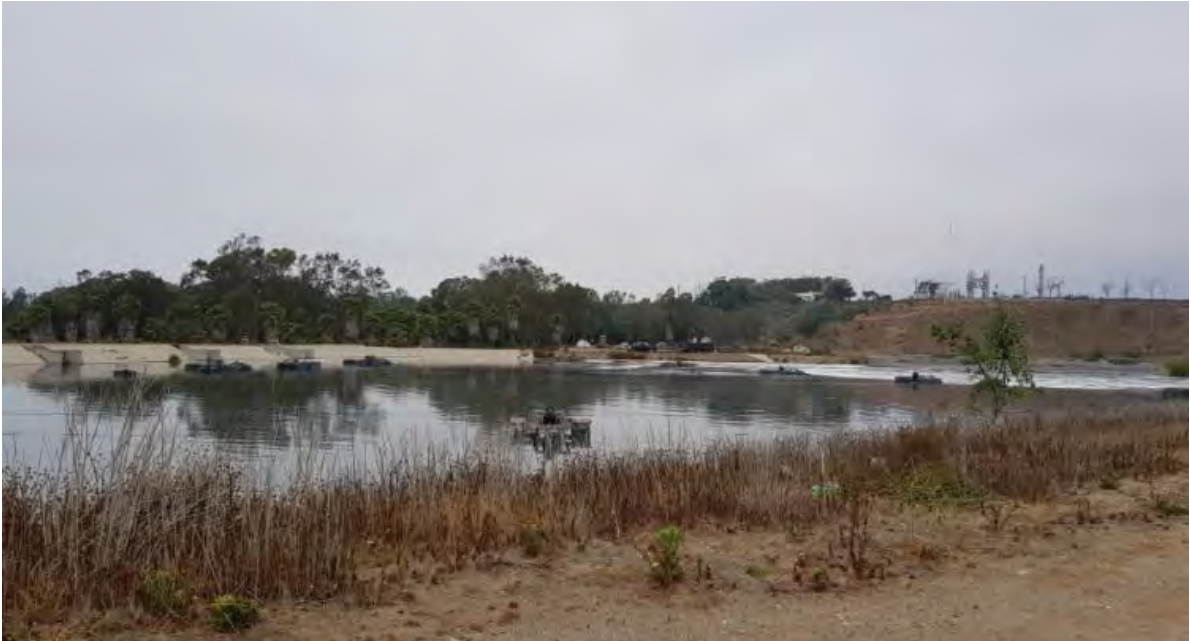
Figure 3-10. Overview of the lagoon system at SAB WWTP.
