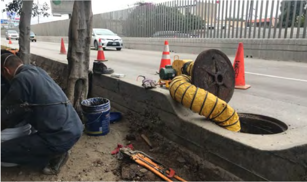
Figure 3-4. Junction box repair at International Collector
