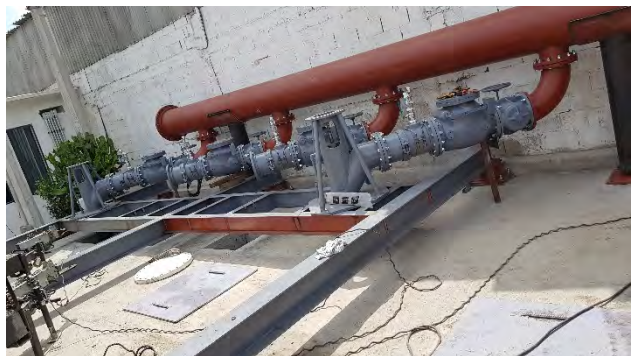
Photograph 8: Pump 2 out of commission, open pipe to have valve replaced
