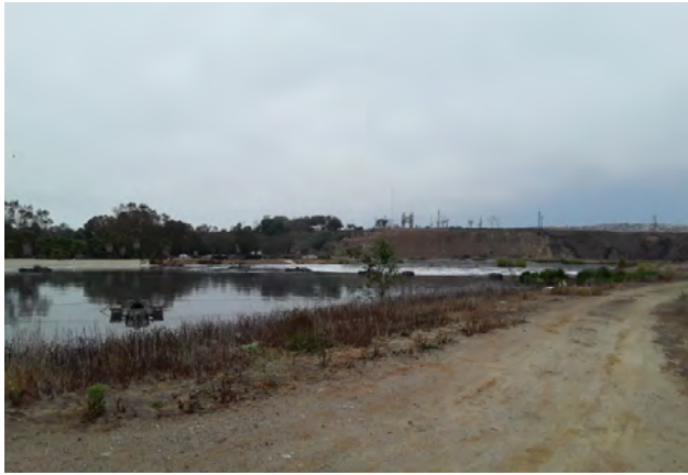
Photograph 19: biological lagoon with non-operational aerators
