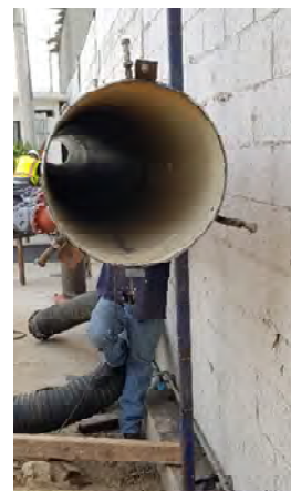
Photograph 12: Welding of new manifold pipe for low flow pumps
