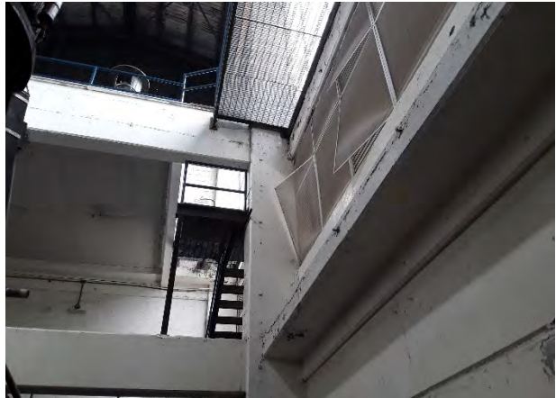
Photograph 26: PB1a Building, interior wall
