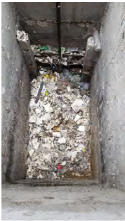
Photograph 51: Inlet box filled with trash
