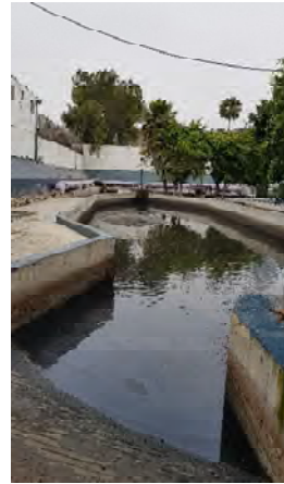
Photograph 2: Sedimentation Channel
