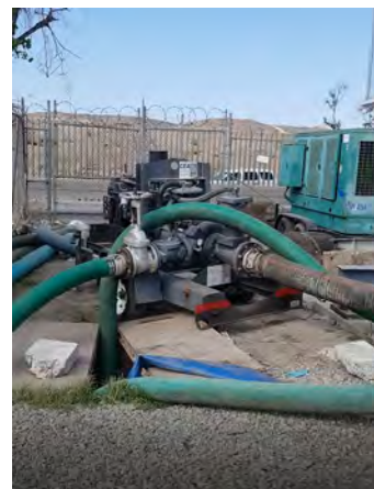
Photograph 6: Temporary pumping to International Collector
