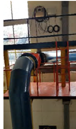
Photograph 10: check valve setup at lift station
