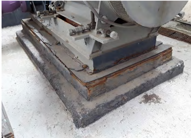
Photograph 25: Old pump train No. 1 concrete base
