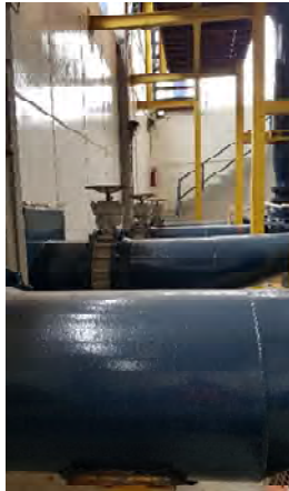
Photograph 13: discharge piping section
