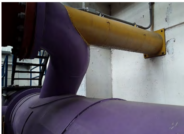
Photograph 23: tie-in to effluent manifold
