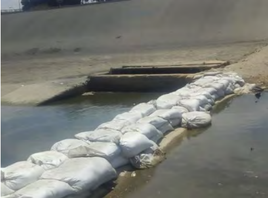
Figure 3-2. View of PBCILA Intake along with temporary berm efforts
