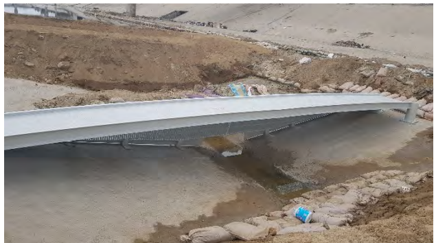
Photograph 10: new dry-weather rack installation at V-notch channel
