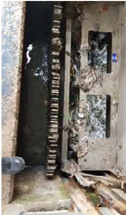
Photograph 49: Trash rack for screens
