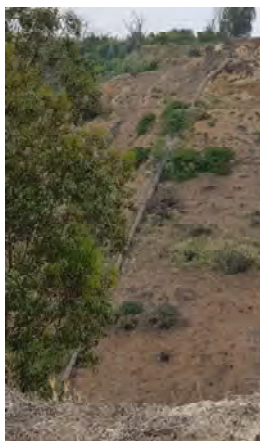
Photograph 23: discharge piping section
