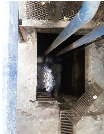
Photograph 46: sump pump setup
