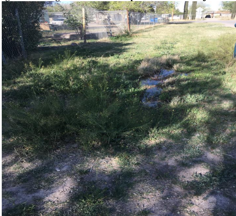
Fig. 14. Standing surface water in septic drainfield in Bejar Estates
