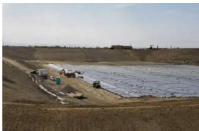
Installation of geomembrane liner
