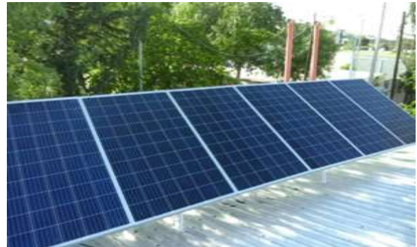
Installation of solar panels on the roof of EcoCasa
