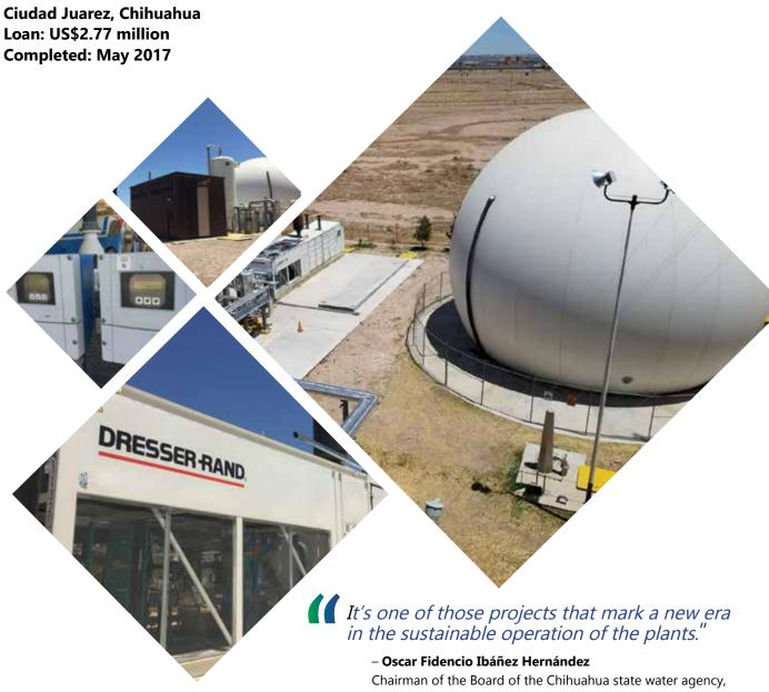
A 1.35-megawatt cogeneration facility was installed to supply up to half of the electricity needed to operate the South Wastewater Treatment Plant (WWTP), which consumed almost 15.46 gigawatt-hours (GWh) in
