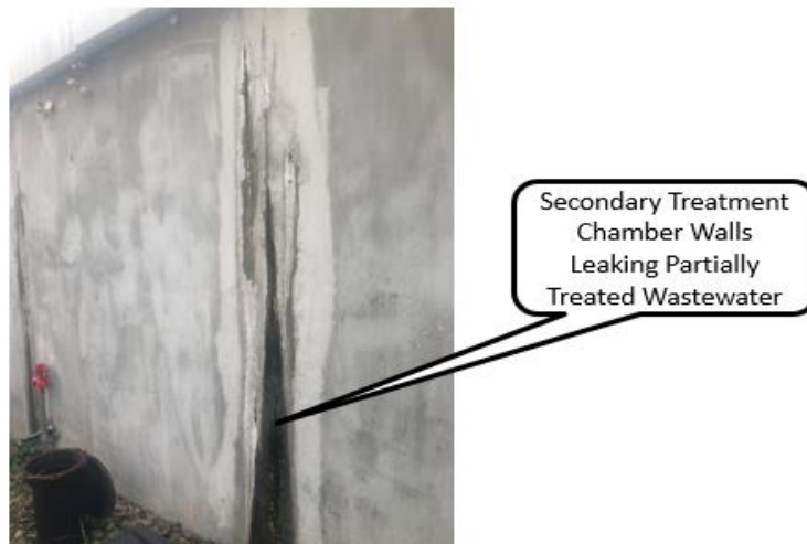
Figure 3 LEAKING BASIN WALLS
