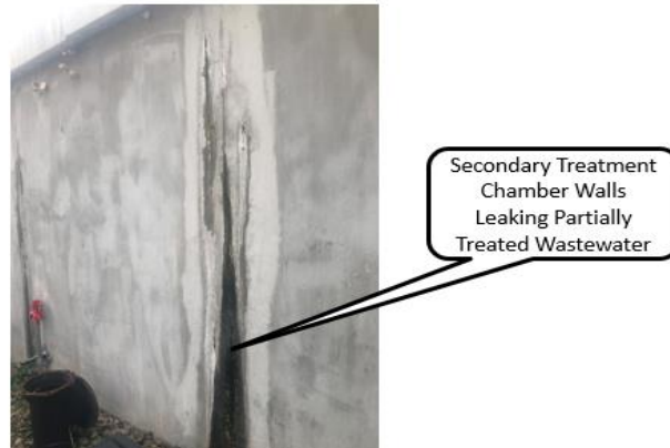
Figure 3 Leaking Basin Walls
