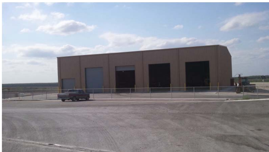
Figure 3 STARR COUNTY SOLID WASTE TRANSFER STATION
