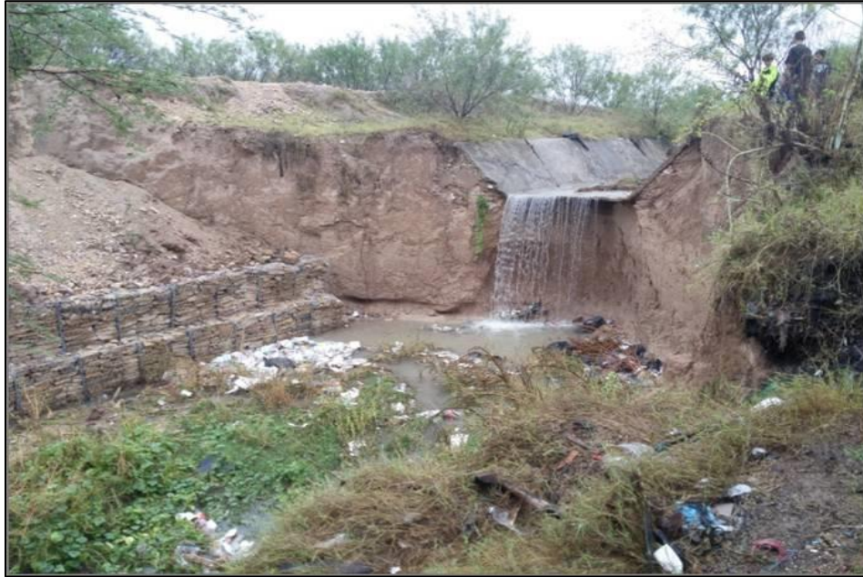
Figure 5 SANTA MARTHA STORM WATER CHANNEL
