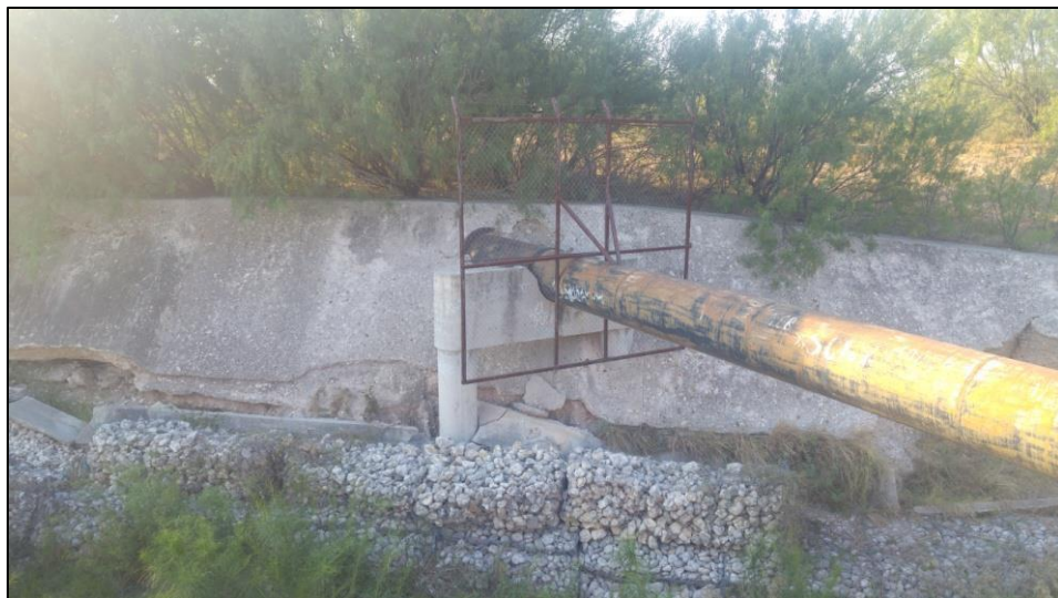
Figure 4 LA MISIÓN STORM WATER CHANNEL AND WASTEWATER FORCE MAIN
